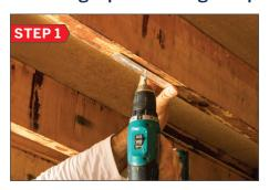
Fix the Optimo straps to the timber joists no greater than 500mm swivelling them so they run parallel to the joist to leave access to the cavity free to install the insulation. Secure the strap with either screws or nails. Either a hammer and nails or drill and self-tapping screws can be used.
