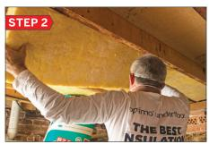
Friction fit Optimo batts tightly between the joists and press in place to ensure there are no gaps between the insulation and underside of floor, joists, or abutting edges (ends) of insulation.
