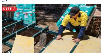
Bradford Optimo™ is most easily installed from above before the floor is installed. Place Optimo™ saddles across joists no greater than 500mm apart so to support batt from both sides, staggering the position of the saddles from joist to joist. Fasten into place using a staple, nail or screw.
