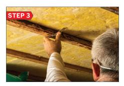
Swivel the Optimo strap 90° so the strap extends into the floor cavity between the joists and bend the strap upwards to support the insulation then tighten the fixing of the strap.
