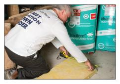
Switch off power at the fuse box. Measure your floor joist spaces. Usually 450mm centres or 600mm centres. For 450mm centres use 415mm wide batts. For 600mm centres use 565mm wide batts. Trim batts with knife if too wide.
