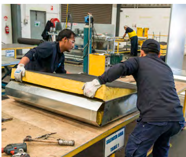
Bradford Ultratel installed inside the baffle frame
