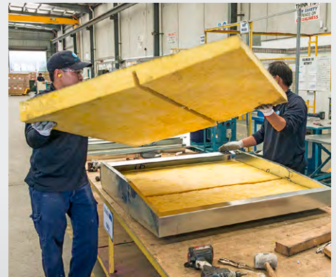
Second layer of Bradford Ultratel installed in the baffle frame
