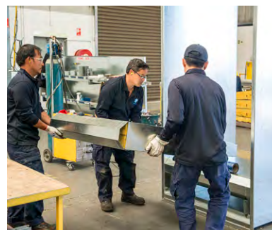
Acoustic baffle installed inside the silencer frame
