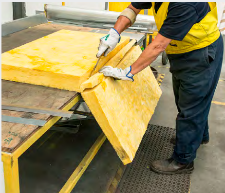
Bradford Ultratel shaped to fit the acoustic baffle frame
