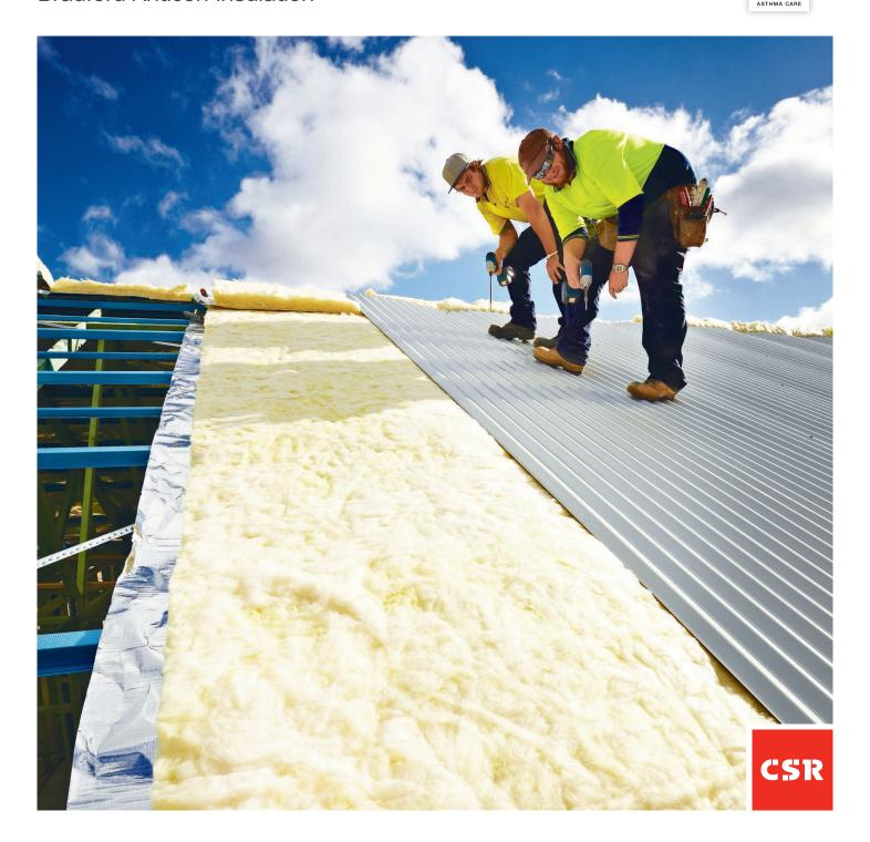
Insulation is proven to be one of the most effective ways of controlling temperature, reducing unwanted noise and mitigating condensation risk in a home. Bradford Anticon combines two components in a single product to provide these benefits. The insulation blanket interrupts the passage of heat and rain noise through your roof. At the same time, the reflective foil restricts the passage of moisture to cold surfaces, reducing your risk of condensation.
