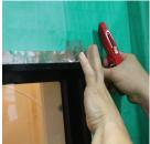
**58% reduction** in air infiltration was achieved when Thermoseal Wall Wrap was installed with overlaps and window frames sealed with tape.
