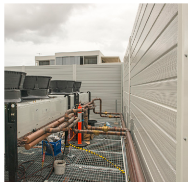
Perforated surfaces face the noise source allowing the sound energy to enter the core and be absorbed
