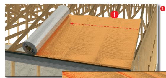
Start by rolling Polyair out across the roof trusses or rafters parallel to the facia. Ensure a 20mm - 40mm sag is created between each truss or rafter and use tape or staples to hold Polyair in place until roof battens are fixed.
