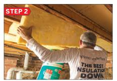
Friction fit Optimo batts tightly between the joists and press in place to ensure there are no gaps between the insulation, underside of floor and joists, or abutting edges (ends) of insulation.
