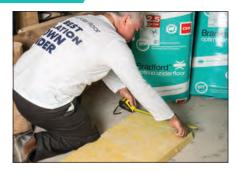
Switch off power at the fuse box. Measure your floor joist spaces. Usually 450mm centres or 600mm centres. For 450mm centres use 415mm wide batts. For 600mm centres use 565mm wide batts. Trim batts with knife if too wide.
