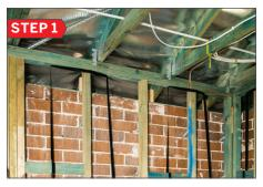
For external walls it is recommended to string to ensure the insulation can not bridge the cavity. Start at the underside of the top plate 75mm in from the vertical stud. Staple polypropylene string to the underside of the top plate. Drop the string to the top of the noggin, tensioning then staple. Run the string towards yourself and turn it to the underside of the noggin and staple. Drop the string to the bottom plate, tensioning then staple.
