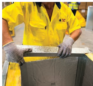
Metal angles installed to complete corners and edges
