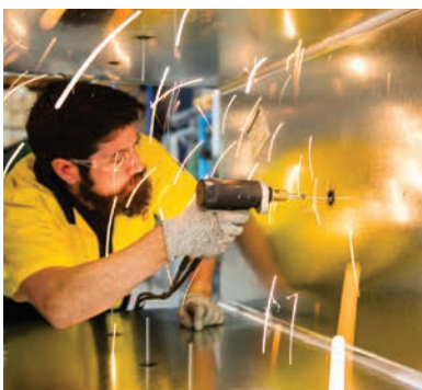
Metal pins welded to internal face of duct
