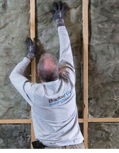
SoundScreen is low allergen and will not shrink, mould, rot or deteriorate. When installed in accordance with their directions, Bradford insulation products are guaranteed for at least 70 years. SoundScreen is also approved by the National Asthma Council's Sensitive Choice® program, making it ideal for the homes of asthma and allergy sufferers.<sup>14</sup>
