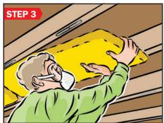
Friction fit Optimo batts tightly between the joists and press in place to ensure there no gaps between the insulation and joists, or abutting edges (ends) of insulation.
