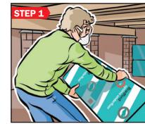
Take enough packs into the underfloor area for the whole job where possible. Start fitting insulation from the furthest point from the underfloor access.
