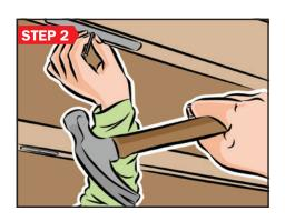
Nail the Optimo aluminium straps to the timber joists every 500mm swivelling them so they run parallel to the joist to leave access to the cavity free to install the insulation. In lieu of hammer & nails you can use drill and self-tapping screws.
