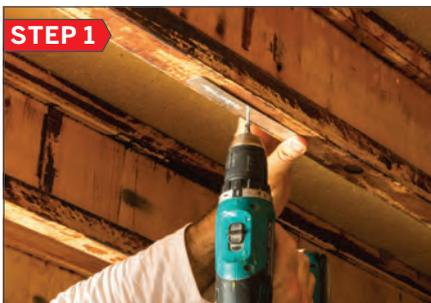
Fix the Optimo straps to the timber joists every 500mm swivelling them so they run parallel to the joist to leave access to the cavity free to install the insulation. Either a hammer and nails or drill and self-tapping screws can be used.
