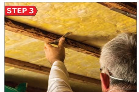
Swivel the Optimo strap 90° so the strap extends into the floor cavity between the joists and bend the strap upwards to support the insulation then tighten the fixing of the strap.
