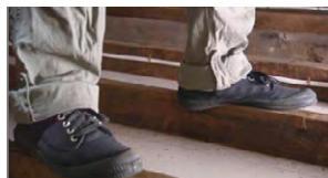
Safety: use joists for footing support
