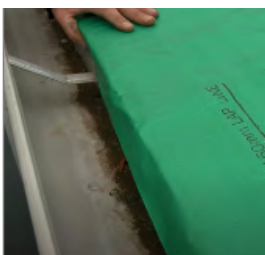
Overlap roof sarking into gutter by up to 25mm
