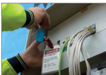
Fixing power sign to meter box
