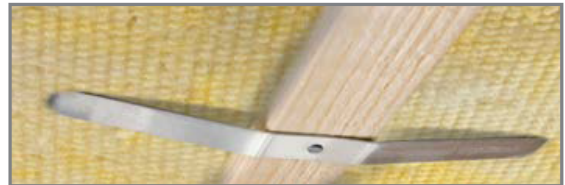
Butterfly clip holding insulation in place
