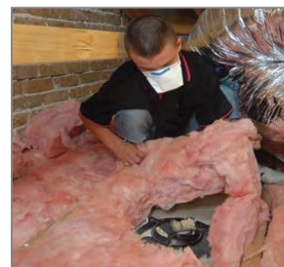
Check table minimum clearances for recessed lumen.
