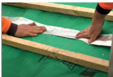
Apply UV stabilized sealing tap if overlap less than 150mm
