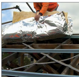
Vertical roll out over horizontal battens
