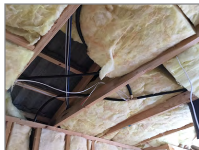
Inadequate number of batts for ceiling insulation. Insulation has been displaced to install wiring and not reinstalled correctly
