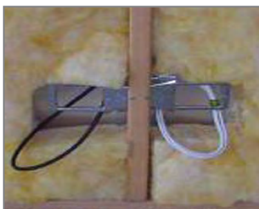
Insulation cut-outs for power points
