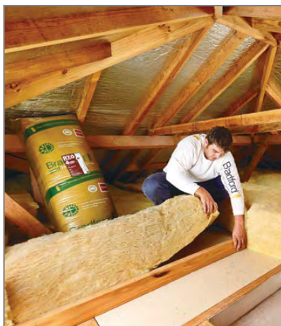
Installing ceiling batts after ceiling linings are fitted.
