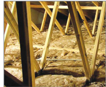
Fully installed ceiling insulation batts - no gaps
