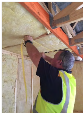
Installing ceiling batts with stringing in method.
