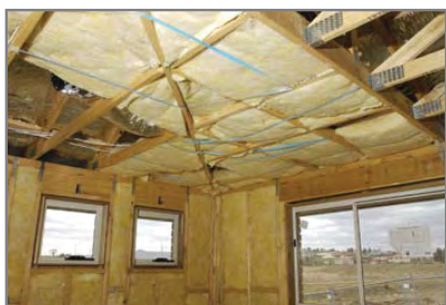
Example of ceiling insulation in progress using stringing
