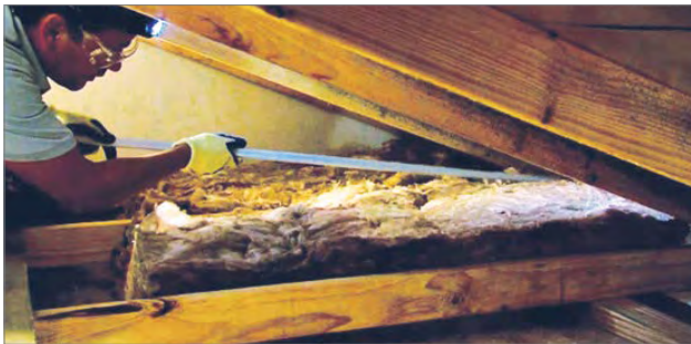
Using non conductive Batt Poker for inaccessible areas.
