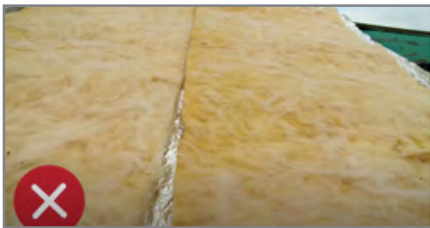
Don't leave gaps - abut blankets together so no facing is visible
