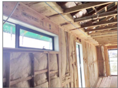
New build - perimeter batts installed.
