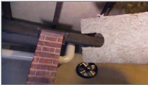
Cutting insulation around under floor services
