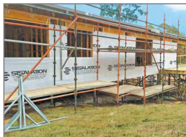
Wall wrap installed prior to windows being fitted
