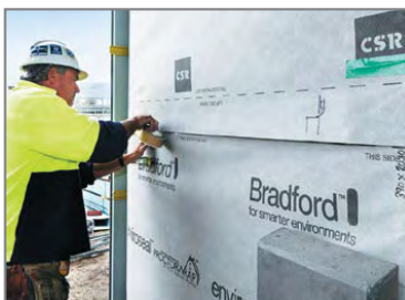
Taping and sealing membrane overlaps
