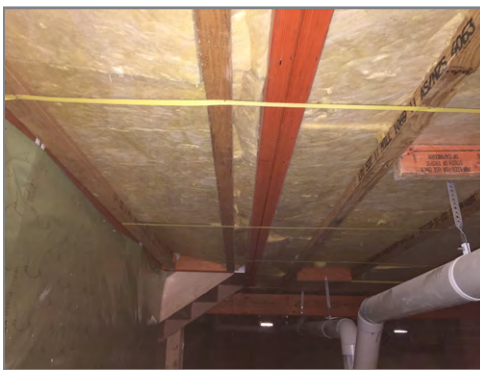
Stringing under floor insulation in place
