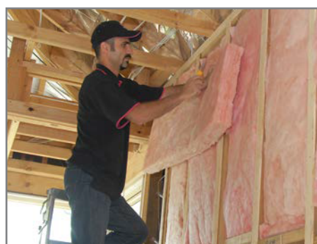
Examples of fitting wall batts
