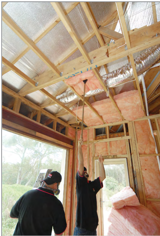
New build - Installing ceiling insulation with limited access due to ducting.
