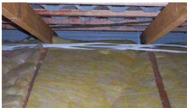
Ensure electrical cables are left on top of insulation along the roof edge. If the tension in the cable does not permit the cable to rest on the top of the ceiling joist if needed use a lesser R-value batt for edge trim.
