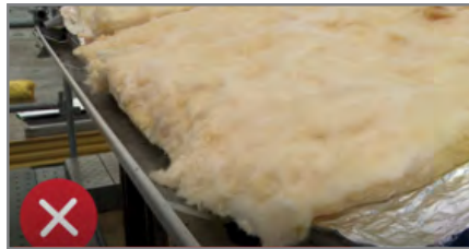
Do not let insulation blanket overhang into gutter
