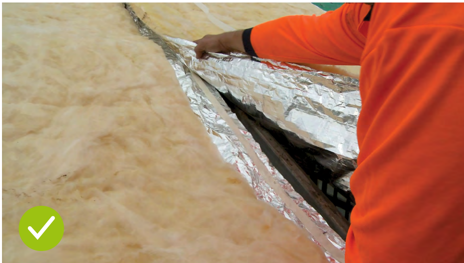
Don't leave gaps - abut blankets together so no facing is visible
