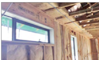
Installing perimeter batts over top plate
