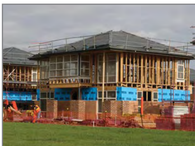
Safety rails fitted for working at heights
