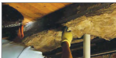
Cutting insulation to install around plumbing services
