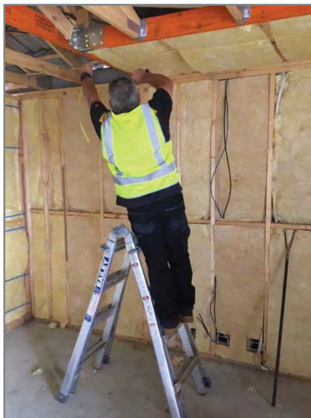
Example of fitting edge batts
