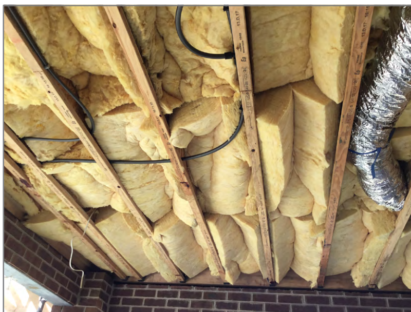
Batts squashed into rafters compromise thermal benefits
