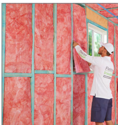
Examples of well installed wall batts
