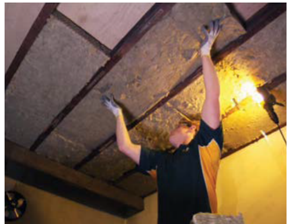
Elevated floor- installing insulation between floor joists
