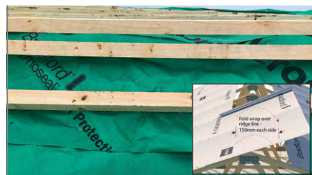
Install sarking from gutter to ridge
