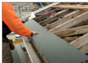
Fixing anti-ponding board
